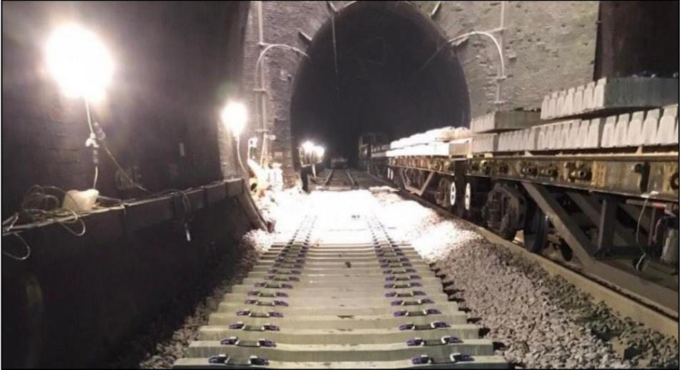
The line was closed between Rugby and Hanslope junction with all services diverted via Northampton. So, opportunity was taken to also complete a significant number of other jobs along the closed section of line which included; rerailing, replacing S&C components, drainage repairs, clearing lineside vegetation, 3500 metres of signalling cable replacement and the stabilisation of a landslip site with 820 tonnes of stone.
